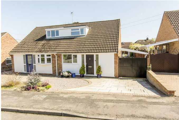
Gravelled front garden with plant beds inset. Paved driveway leading to gated car port and rear garden.
